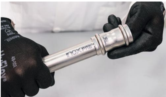
Figure 24 - Inserting pipe into the press fitting
