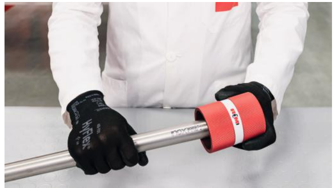
Figure 20 - Deburring the pipe
