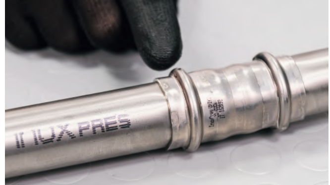
Figure 26 - Checking the press connection
